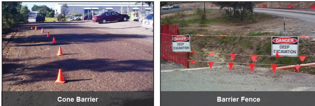
Fig 5.2 Cone Barrier and barrier fence
